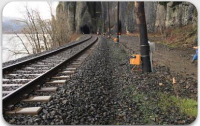
Rockfall Monitoring System
