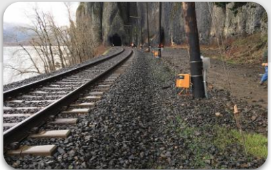
Rockfall Monitoring System
