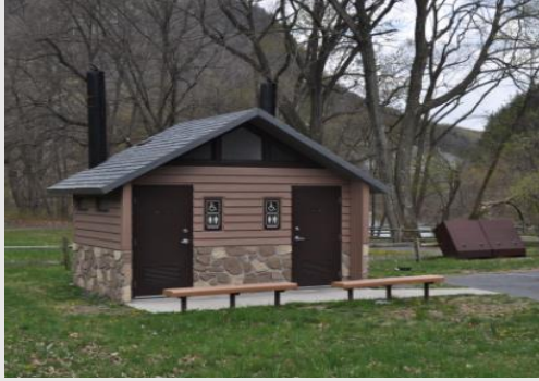
Precast concrete building
