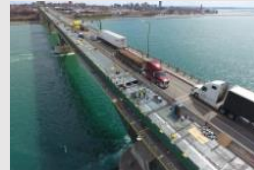
Peace Bridge – Buffalo, NY to Fort Erie, ON
