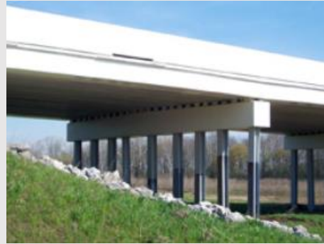
Prestressed box beams
